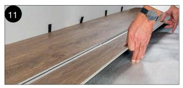
DISASSEMBLING THE LONG SIDE Lift up the entire row in the same angle as you did during installation, then slide the rows apart.
